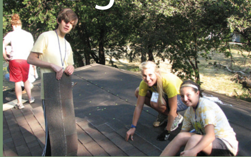
Students reroof one of the project homes.
